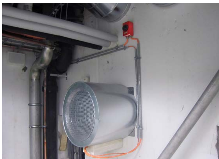
KATKO Firerated switches at Keilaniemi metro station in Espoo, Finland
