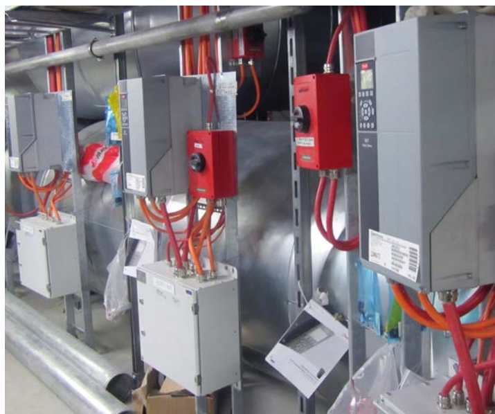
KATKO Firerated switches at Keilaniemi metro station in Espoo, Finland
